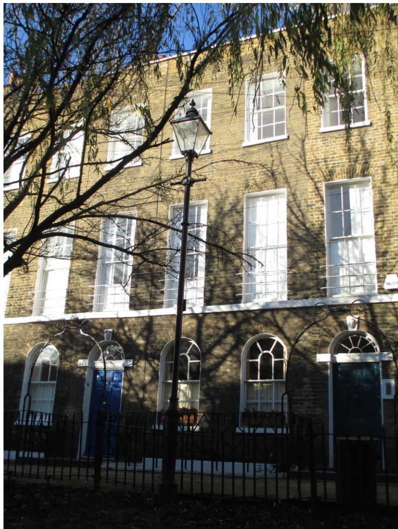
Image 2 - View of front elevation of site
