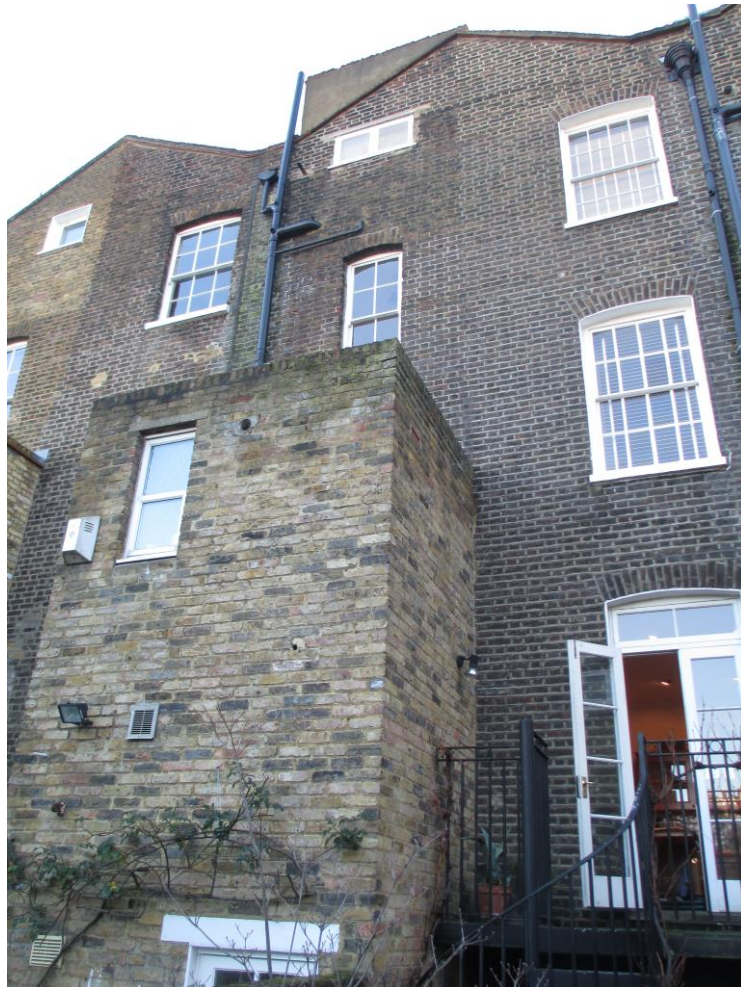
Image 6 – view towards rear elevation of no. 51 from rear garden
